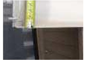
Cut off the trailing-edge up-stand, and cut a one-inch notch out of the louver with the angle grinder as shown.
