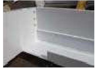
Measure five-and-one-quarter inches along the face of the side gutters and mark. Follow the picture instructions to make a flap that will bend around the corner when you put the gutters together.
