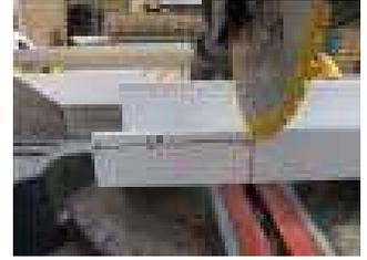
Mount the gutter by screwing it onto the back beam. Repeat the procedure for the front beam.
