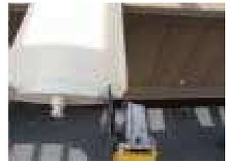
When installing the two louvers next to the motor, roll in the far end first, ensuring that it is in its pocket. Then roll in the side next to the motor. You may have to operate the motor to get the louver to move past the motor arm and sit correctly in the pocket.
