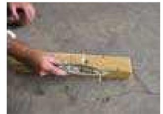
Use the special field tool to hammer on the new retention clip.
