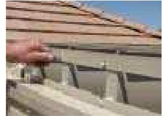
The two louvers next to the motor have to be notched so that they will clear the motor and electrical connections.
