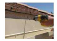
You can also pre-drill the center of the beam with a quarter-inch hole and open it up to seven-eighths inches with a multi bit, and fasten through the back wall of the beam using a three inch screw. You can then cap that hole with a plug. With a wall mount situation, you can pre-drill the bottom three inches of the beam and cover the hole with the gutter.
