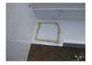
Put side gutters in place and silicone behind the flap before screwing it in place.
