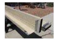
Measure between the front and rear beams to get the side gutter measurement. Deduct three-eighths of an inch from that measurement to ensure that the gutter clears the flanges of the front and rear gutters.
