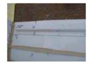
You will never have more than a four inch gap on each side, because at that point you can fit another louver in. Use the measuring chart for calculating the optimum width. Or, layout the pivot strips end to end on the ground, to determine how many louvers will fit within the framework.
