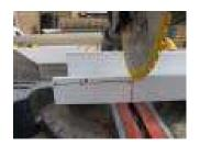
Mount the gutter by screwing it onto the back beam. Repeat the procedure for the front beam.
