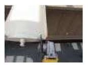
When installing the two louvers next to the motor, roll in the far end first, ensuring that it is in its pocket. Then roll in the side next to the motor. You may have to operate the motor to get the louver to move past the motor arm and sit correctly in the pocket.
