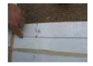
The pivot strip must have factory ends butted together to ensure proper spacing of the louvers. Screw pivot strip in place with five-sixteenth inch screws.
