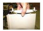
After cutting the louver, use a rubber mallet to pound the end cap on.
