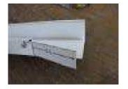
Put silicone sealant in the bottom of the front and rear gutters before putting the side gutters in place.
